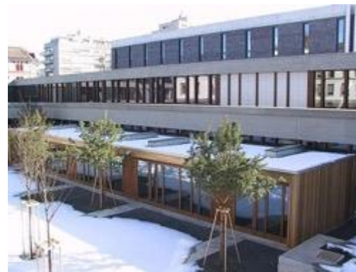
Burggraben Cantonal School
