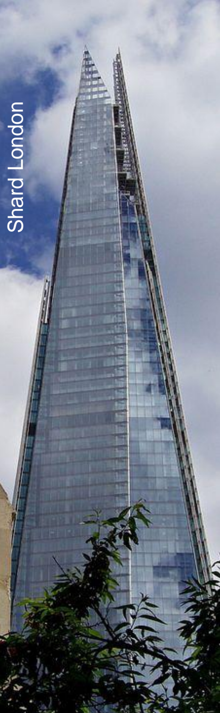
Roche Tower Rotkreuz
